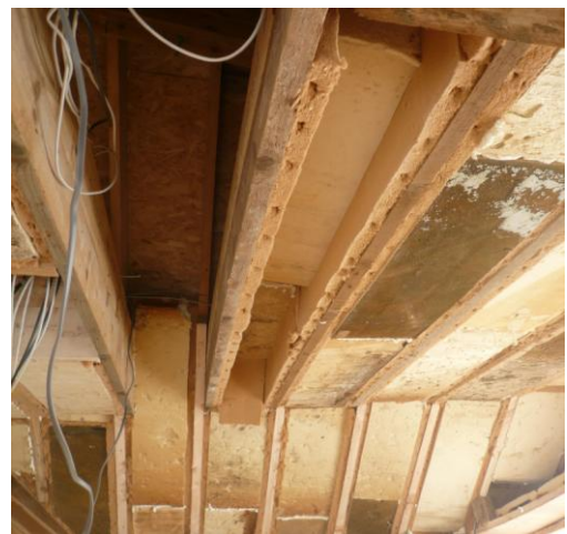
40mm Wood-Fibre Insulation Lining Rafters and Joists with Salvaged Insulation Sandwiched in Between
