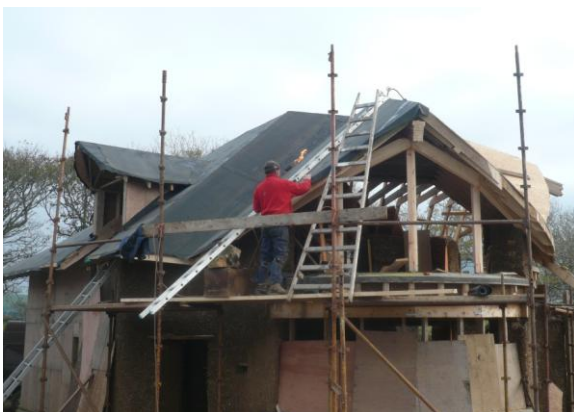
Applying Bituminous Felt to Roof
