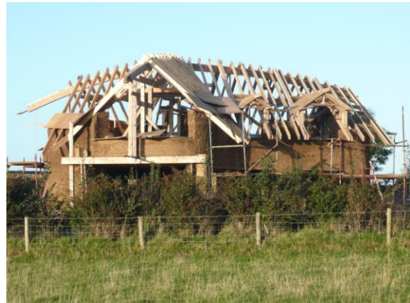
Mud and Wood House Roof
