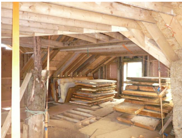
Freezer-Unit Insulation Ready to be Installed
