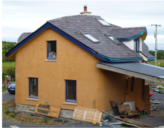
Hemp-Lime Render Applied to Boards
