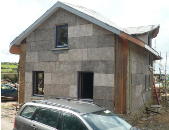
Salvaged Wood-Fibre and Cement Boards
