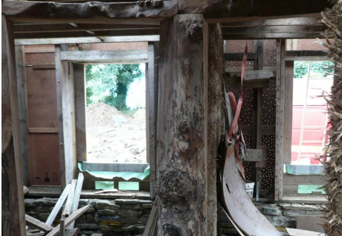
Salvaged Plywood – Note Hundreds of Tiny Holes Drilled in Plywood Sheet on Right-Hand-Side
