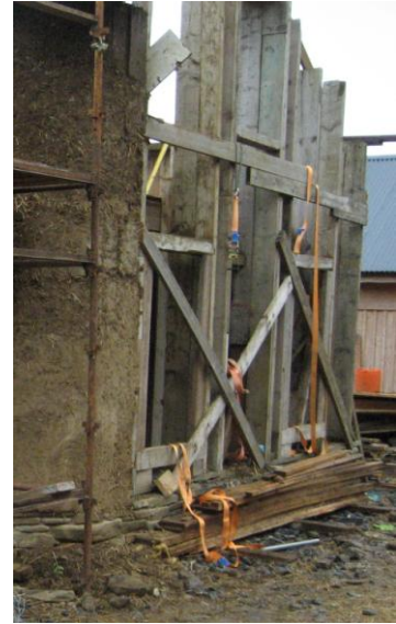
470mm Deep Timber Studs
