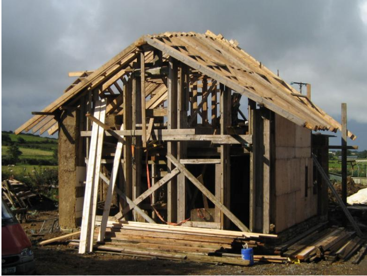
Timber Frame Wall Made from Small Timber Sections
