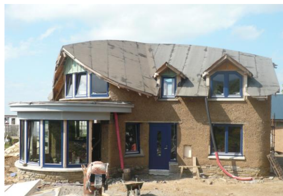
Felt Roof Covering Bought Plenty of Time to Find Good Quality Slates
