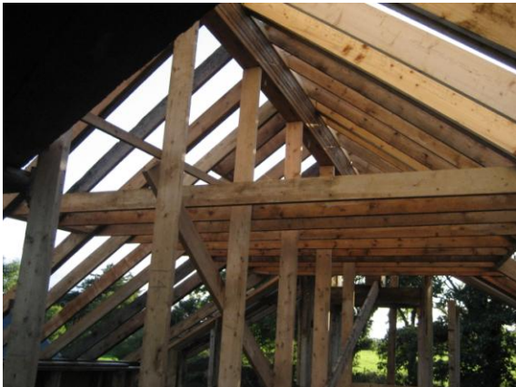
Salvaged Roof Timbers
